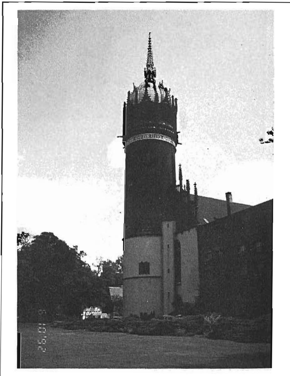
The lower section of the tower consists of plastered masonry. The plaster, which contains cement, was renewed only a few years ago. The upper section consists of sandstone squares and sandstone ornaments. The surfaces are badly soiled and in the rain-protected areas in particular there are thick, black crusts of dirt as shown by the next photograph.
