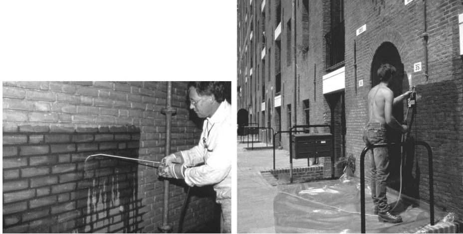
Figure 14: Right product and wrong way of application, top down method (left). Right product and right way of application, bottom up method (right).
