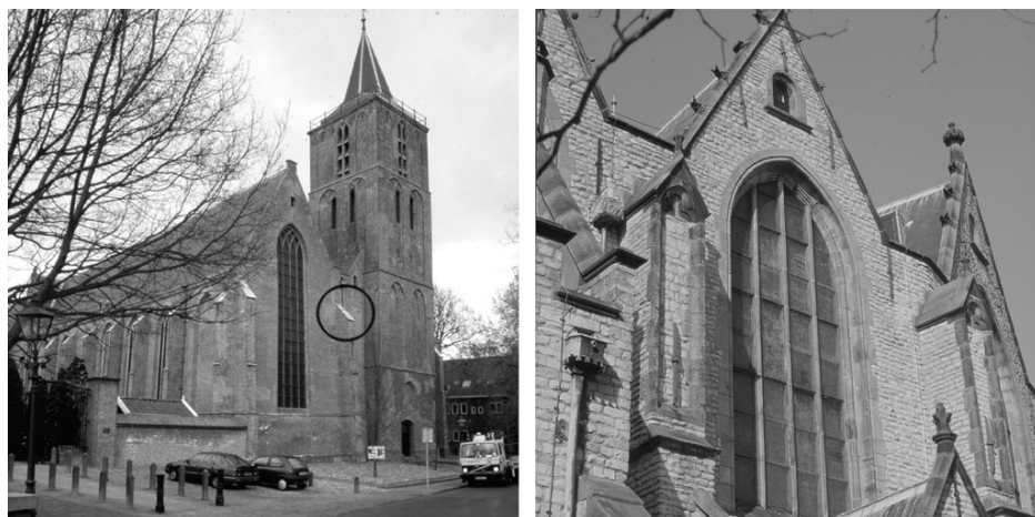
Figure 10: Using architecture to prevent water penetrate into the upright course of the buttress
