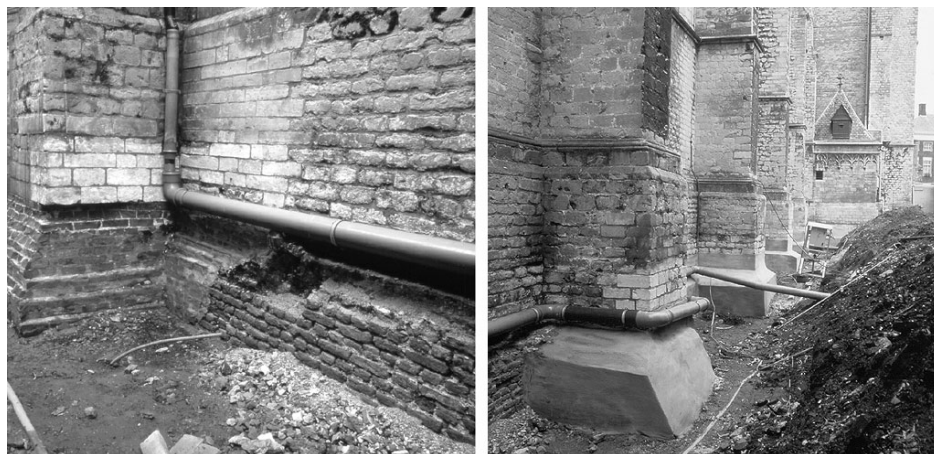
Figure 13: The brickwork under the stone absorbs water easily (left). Protecting the brickwork by plaster and after that by foil (right)
