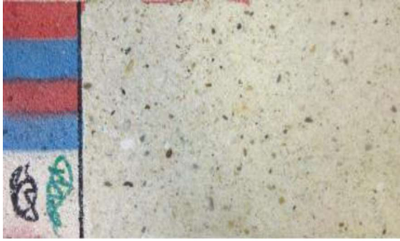
Fig.4. Surface aspect after the first cleaning operation
