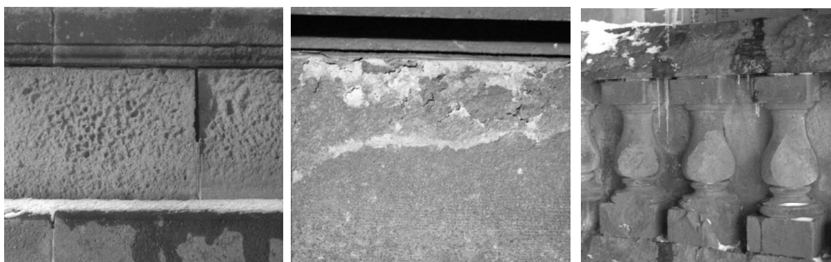
Fig.3. Freezing damages to the stones
