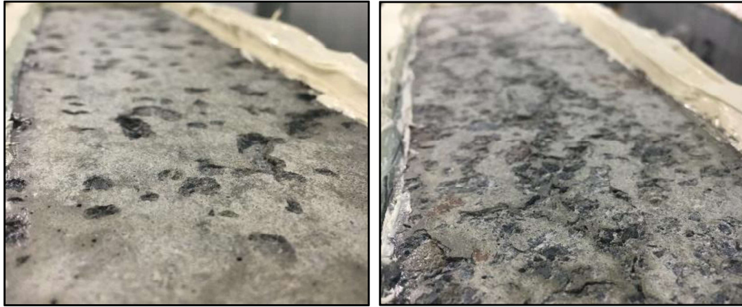
(a) RCIN (b) RCIS Fig. 3. Scaling of RC specimens after 30 cycles of freezing and thawing.
