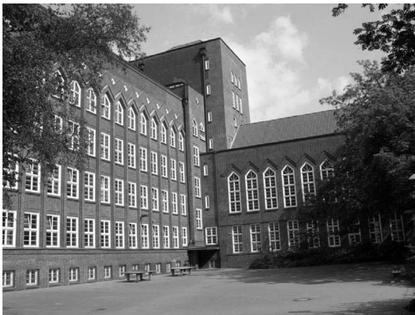
Figure 6: Typical architecture of buildings made of peat moss fired clinker in the Hamburg area. The practically non-absorbent, very hard clinker is typical
