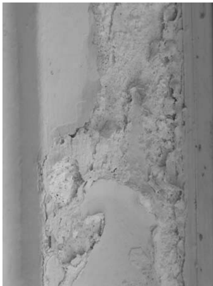
Figure 7: Damage caused by moisture in an interior area of the school building shown in III. 6 – the extent of the damage indicates the magnitude of the quantity of moisture penetrating into the building
