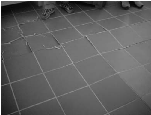
Figure 1: Damaged pavement of the upper floor apartment visited
