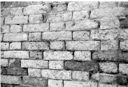
Figure 1: Salt efflorescences on bricks surface
