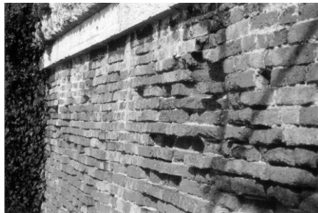
Figure 2: Weathering from marine spray on brick surface
